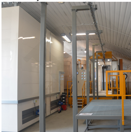
Suspended chain conveyors
